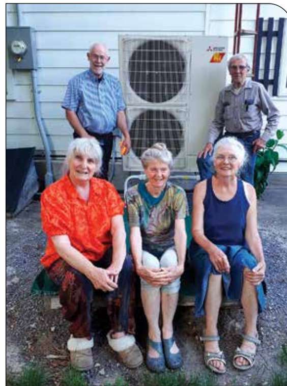
Pictured above are members of one of Climate Network Lanark's very first Concierges — groups that meet regularly to support each other in finding and implementing the best ways to cut greenhouse gases in their home. The next phase of this fantastic program is starting up and seeking new members!
